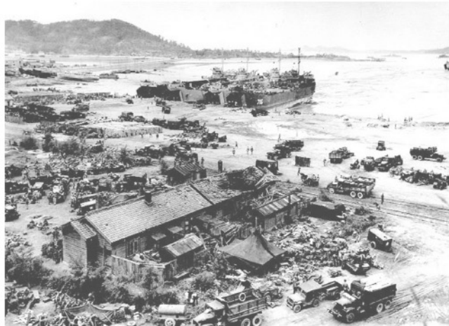
Four tank landing ships unload men and equipment at low tide on Inchon's Red Beach one day after the initial landings there in September 1950 during the Korean War. The authors see this landing as a perfect example of how amphibious operators need to be flexible.
